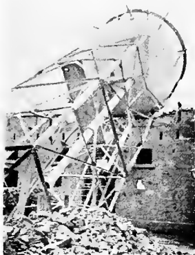
WIRELESS STATION, BAGHDAD. Destroyed by the Huns.
